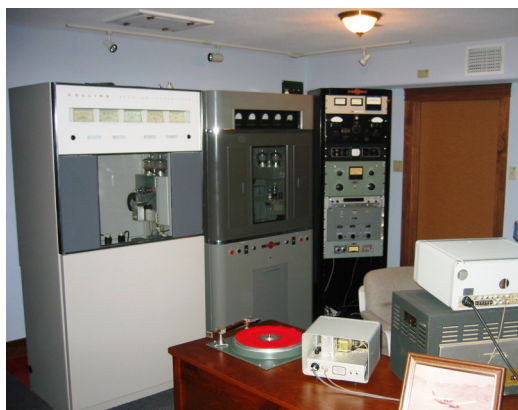
Figure 1. Studio equipment installed, tubed and ready for control and audio cabling
