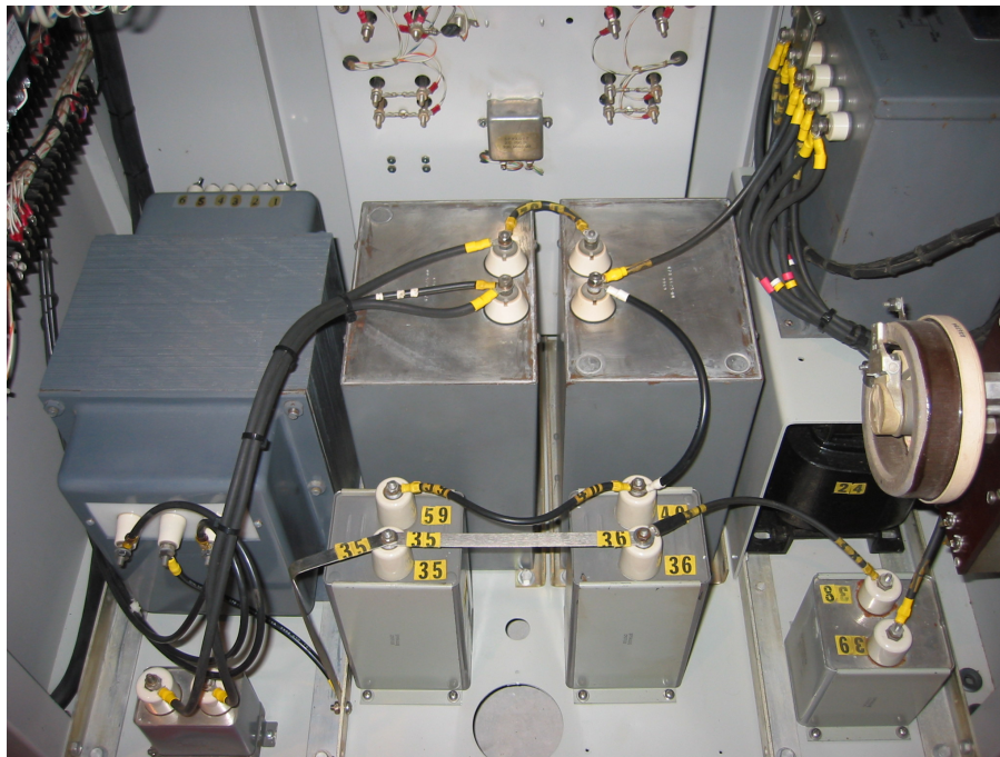
Figure 4. High voltage bottom compartment of the 20V-3 showing placement of the harness and component wiring
