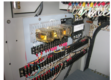
Figure 5. Control panel added in the 20V-3 interface area
